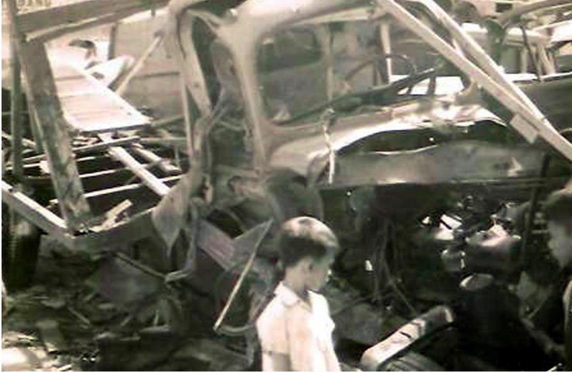
First photograph shows the holes made in the outer and inner walls of the house connected to Ahn Hoa hotel. Destroyed truck was thrown against the building wall on the other side of the narrow alley. (Photos by John Lewis).
